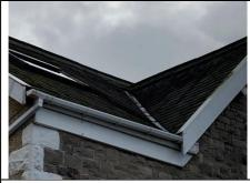
The roof is pitched, with a large dormer feature at the front, and covered in natural slate, which appears to be of local type. The roof has been re-covered in the past from what could be seen internally (not recently). So far as could be seen from ground level, some repairs have been necessary, with re-fixed slates just apparent in places, although not unusual for a roof of this type and age.
