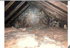
The second floor is part in the roof area, with outer sloping ceilings beneath the roofline. There is a hatch in the top floor landing ceiling, which enables a view into the upper part of the roof space. This revealed the roof of traditional construction. Slates have been laid over conventional roofing felt, which indicates that whilst it has been re-roofed, it will have been some time ago.
